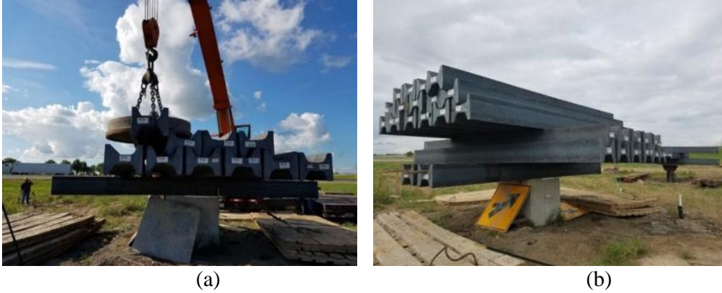
Figure A.17. Photographs of (a) beam blanks being placed at the top of the north drilled shaft, and (b) an axial load of 352.40 kips placed at the top of the North drilled shaft (Photo courtesy by the author).
